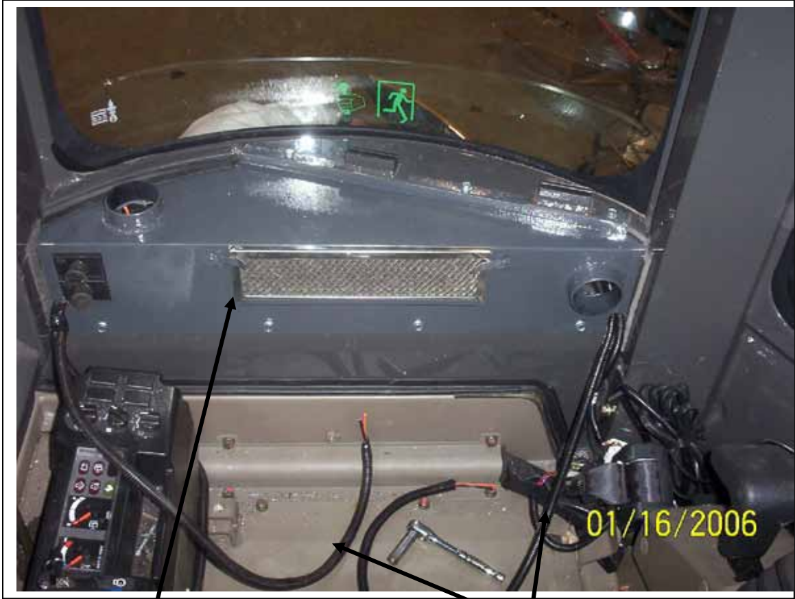
Evaporator cover in place.
