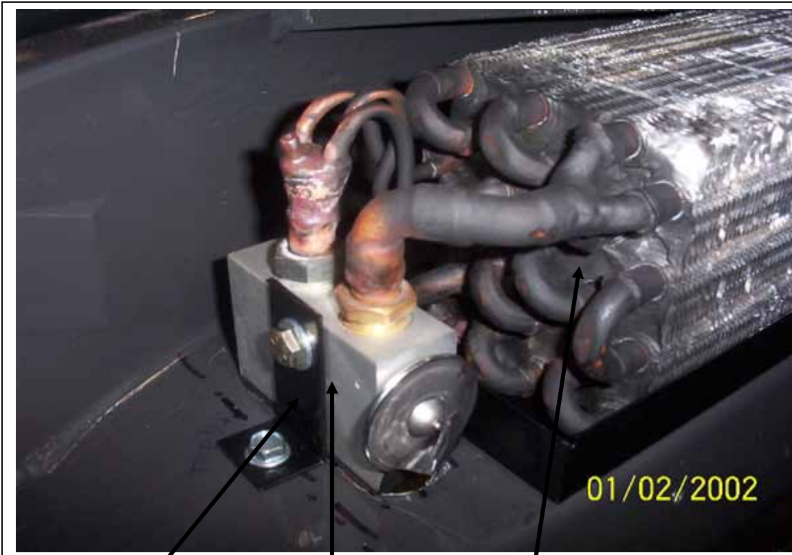
Install evaporator coil and drain pan.
